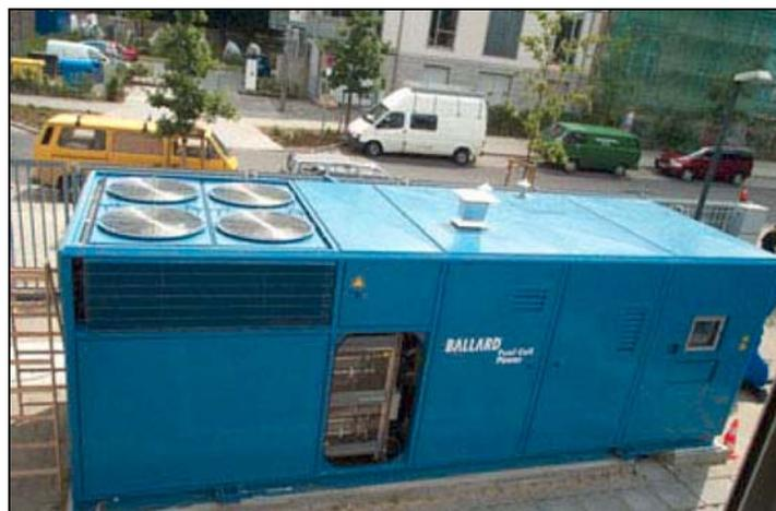
**Figura 7** Impianto Ballard 250 kW, Bewag Treptow Heating Plant, Berlino
